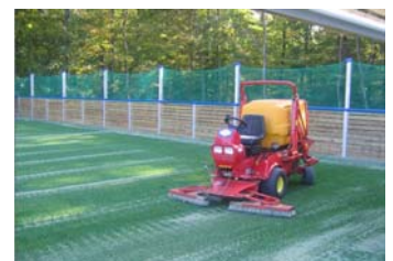
Finally, the rubber-sand mixture is distributed over the artificial turf providing resilience and stability.
