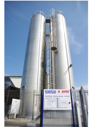
New production plant of Sekisui Alveo in Bad Sobernheim / Germany.
